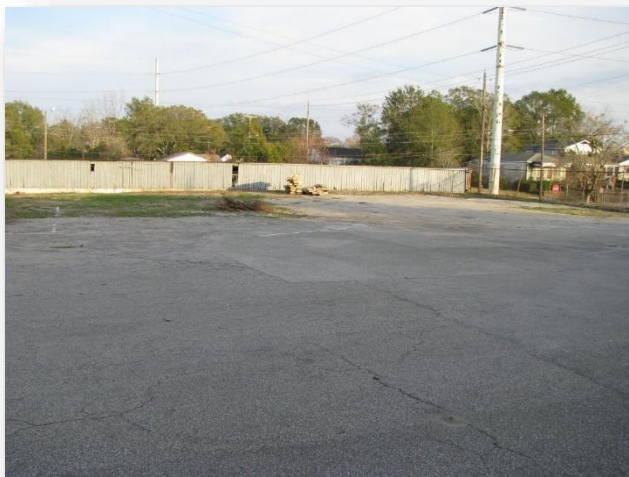
DREAMS parking lot pre-construction
